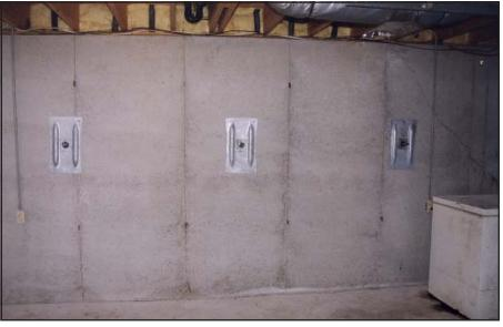
install through poor surface soils and embed in solid lower layers. Special brackets then attach the foundation footings to the anchors.
