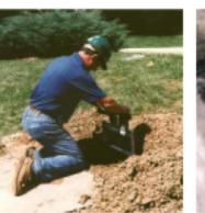
Anchoring points are determined to remedy the damage. Pilot holes are drilled at a descending angle.
