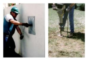
**4** Final adjustments are set on the anchor rods to maintain the new wall position. Anchor holes are refilled, compacted and sod plugs replaced. It's almost invisible!
